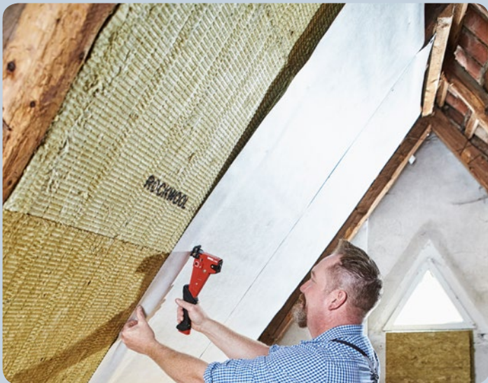
Fastening down sheeting in a loft.
