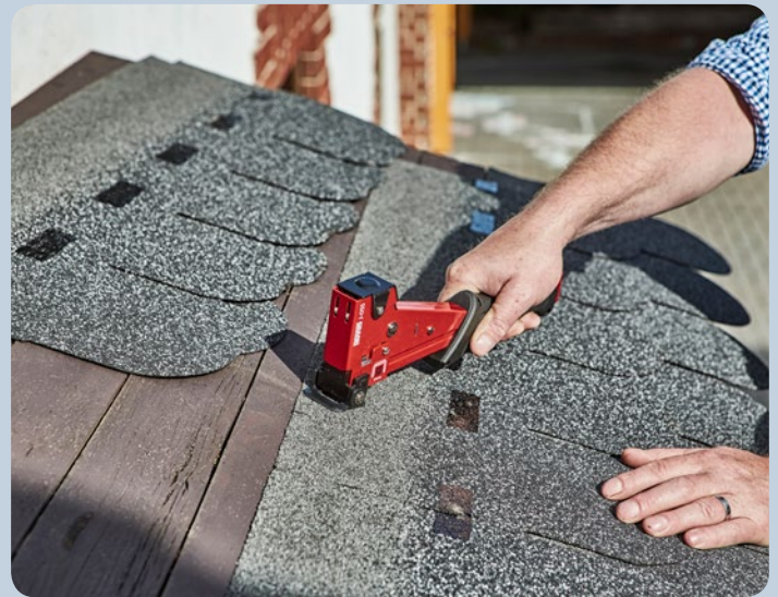
Rapid fitting of bitumen shingles.
