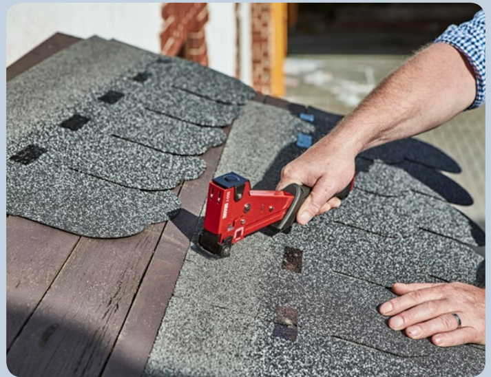
Rapid fitting of bitumen shingles.
