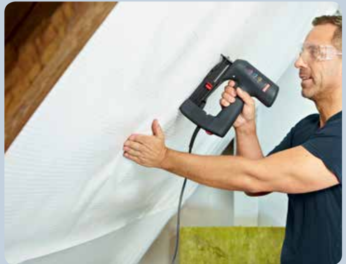
Fastening down sheeting in a loft.
