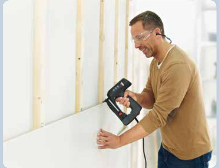
Fastening of tongue-and groove boards with clips.
