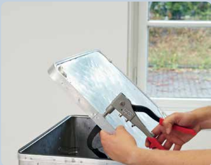
Riveting can be even used for reliably repairing firm materials, like aluminium.
